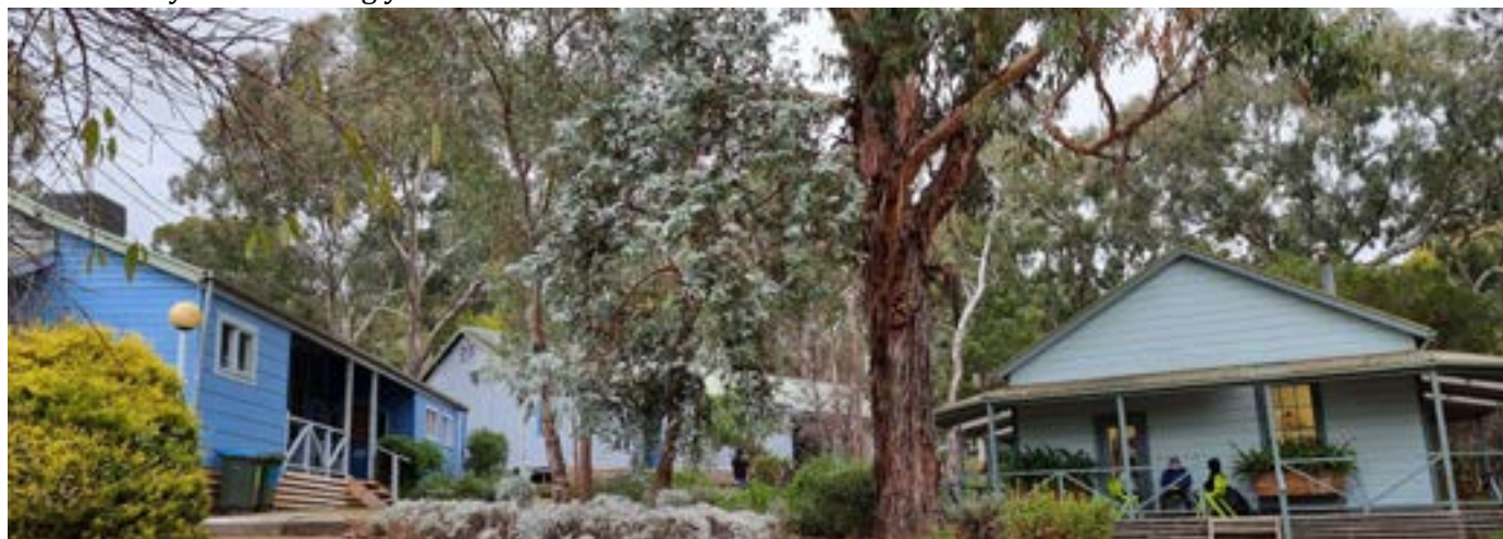
OSHC, Music Room and Hub have been repainted
